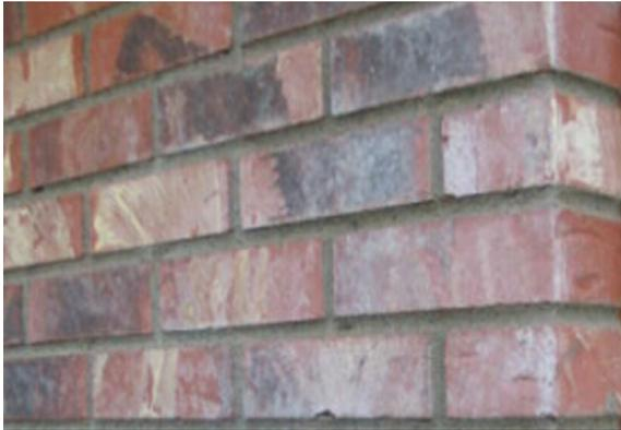
Figure 7 Calcium carbonate on face block work
