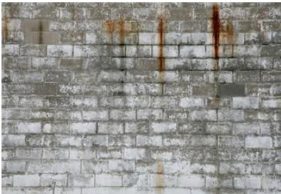
Figure 8 Acid burn on concrete masonry block
