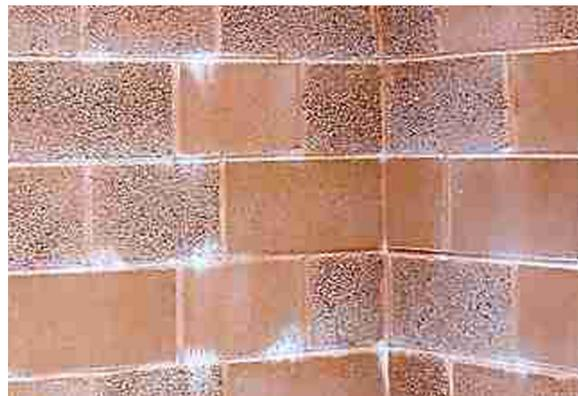
Figure 5 Efflorescence as seen on block faces (a)
